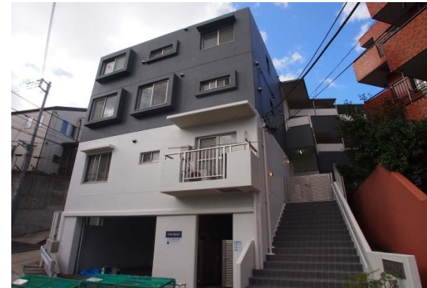
After value-adding renovation
